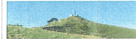
View to Telecom Tower from Upper Bush Cluster
