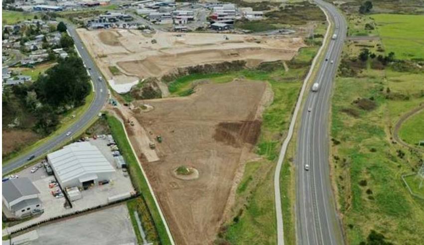
The Crown Road development site during the earthworks phase last September.
