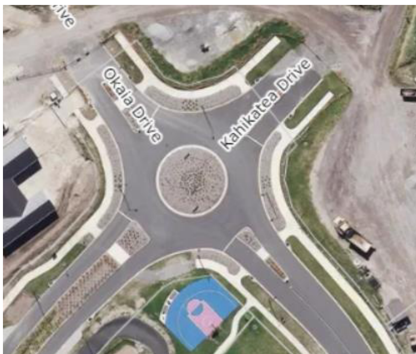
Figure 17: Aerial View of Okaia Drive / Kahikatea Drive Roundabout Intersection
