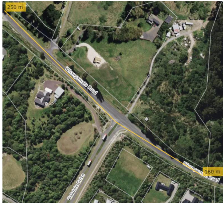
Figure 22: Aerial View of Oakdale Drive / Whangamata Road Intersection
