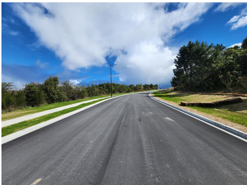
Figure 7: Kahikatea Drive carriageway extension
