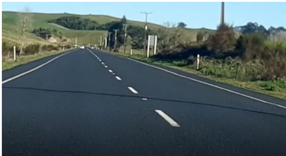
Figure 29 Typical Cross-Section of Pohipi Road between Wairakei Drive and Whangamata Road
