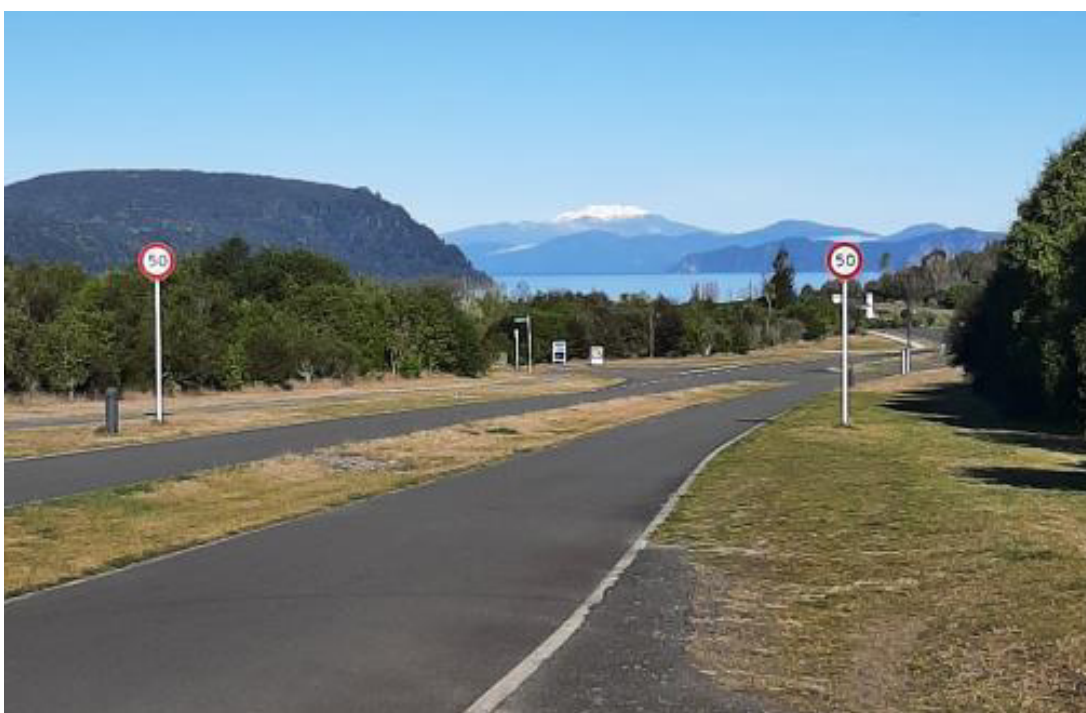
Figure 9: Oakdale Drive northern end - at the intersection with Whangamata Road
